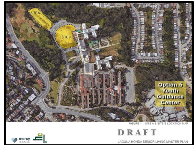
FIGURE 1 : SITE A & SITE B LOCATION MAP A Toxic Site?: Mercy Housing’s draft “ Master Plan ” for senior housing includes three potential site options: “Site A” and “Site B” on the northwest campus (upper left in photo), and “still to be determined” “Option 5” on San Francisco’s former Youth Guidance Center grounds.”
