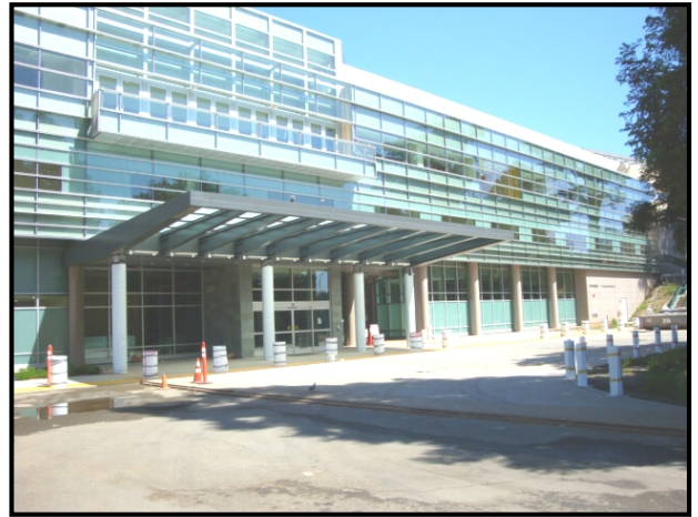
Shortly following excavation, the Health Commission was told in June 2004 of a $25 million cost overrun; in five short years, overruns skyrocketed to $183.4 million, largely due to “change orders.” Where was the CGOBOC?
