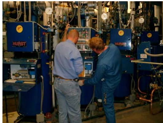
Testing New Boilers
