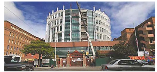
The new SFGH facility never included outpatient dialysis services, even in space vacated in other buildings on campus that will become available.
